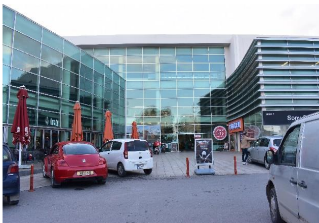
Fig 19: Showing the parking lot of Lemar
